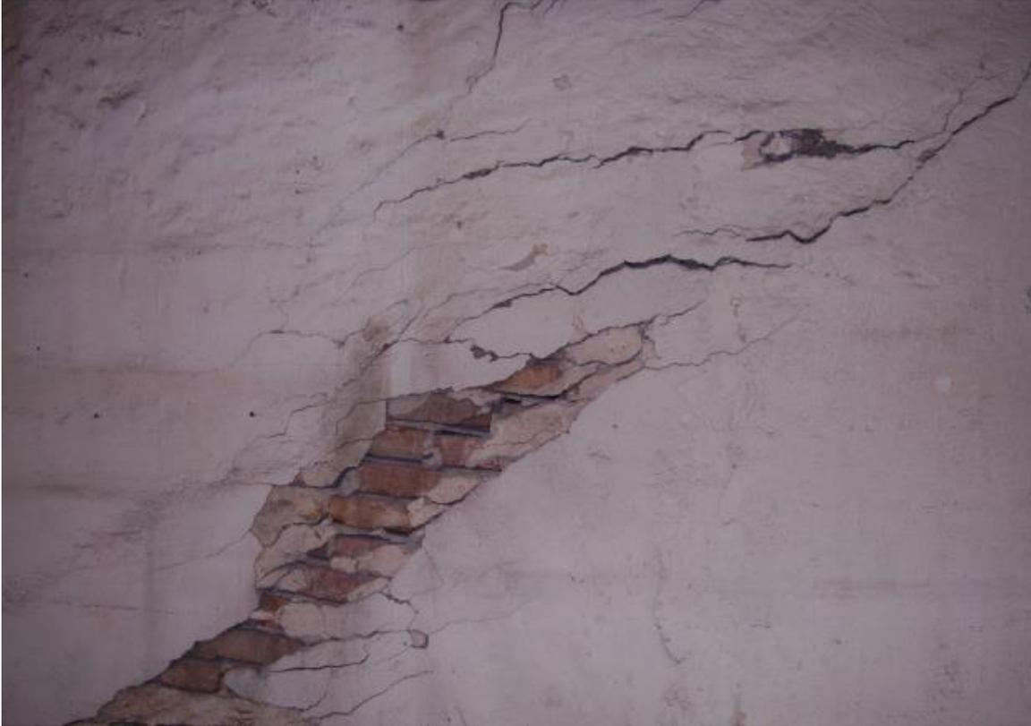
Picture 8. Cracks in a basement wall because the ground beneath the wall had sunk, and the wall was not supported by piles. When we drilled holes in the wall, we found that it was about 0.3 meters between the ground and the underside of the wall. To ensure the function we built a beam construction, resting on piles down to bedrock, outside of the wall. The design did both keep the wall upright and took over its load supporting function.
